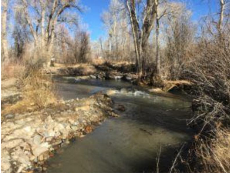
(caption) After restoration, natural structures help control the river grade between upstream and downstream sections. The river now has a serviceable flood plain that will absorb high flows, and bank erosion is under control. Photo by Jason Willis
